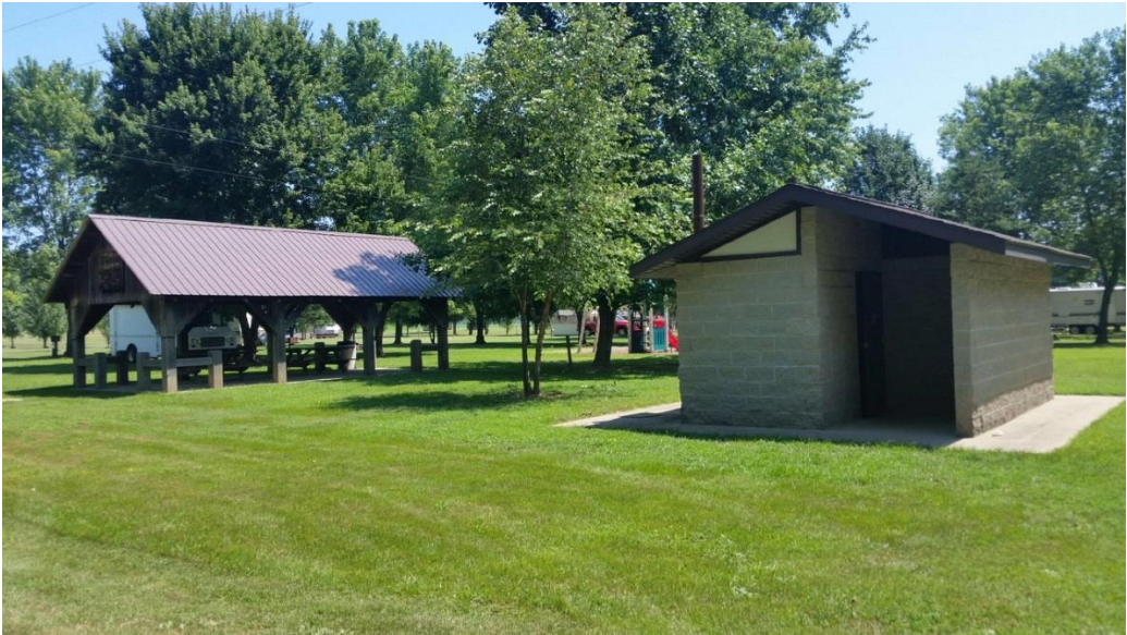
Shelter and restrooms; play area behind
