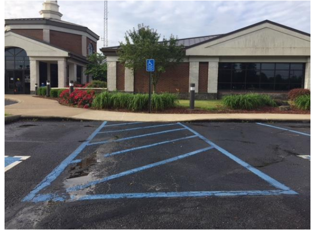
Curb ramp – from Northwest toward Entrance
